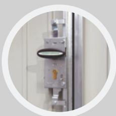
Doors with a built in "Wicket" access door have an additional handle and lock to operate and secure the door. The handle engages and releases twin cable operated latches.
